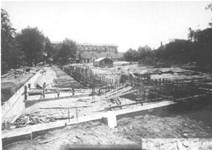
The construction of the Natural Science Building, 1914.
