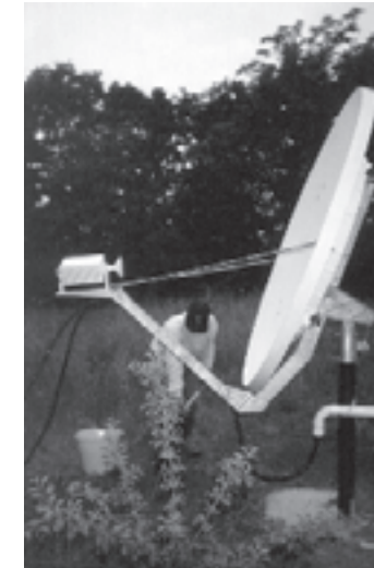
Scott Baird working to install the Ann Arbor USNSN borehole station. The satellite dish provides rapid data transmission.
